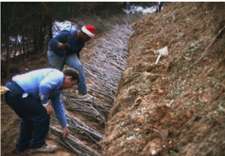
Figure 18-12b Placing live branch cuttings (Note crisscross configuration)
