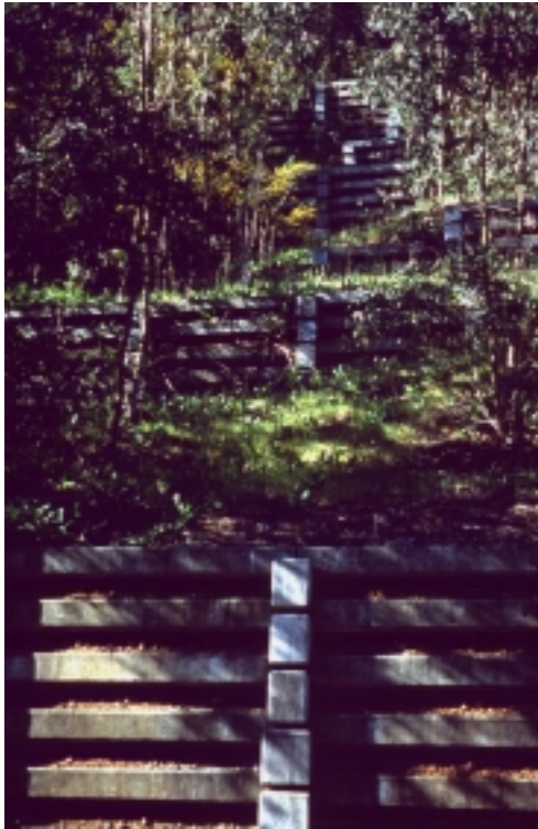
Figure 18-28b Open-front concrete cribwall with plantings in openings
