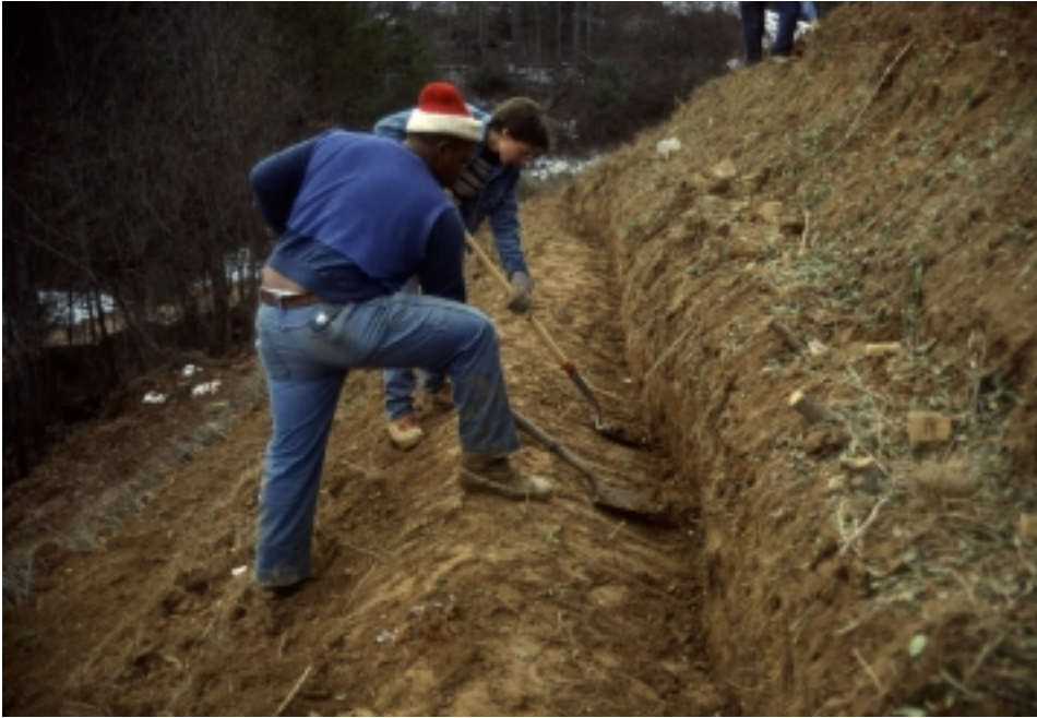
Figure 18-12b Placing live branch cuttings (Note crisscross configuration)
